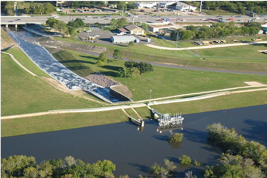
Figure 5 - Barker Dam at Outlet Works during reservoir impoundment
